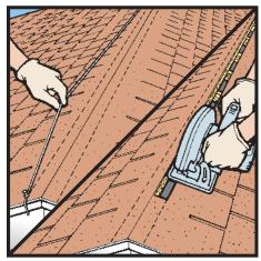
**1.** Measure a 3" slot, 1½" each side of ridge centerline. This allows for a 2x ridge board or smaller. Snap chalk lines the entire length of the ridge. Cut slot with circular saw and clean out debris. Set saw depth so as not to cut roof rafters. Stop slot 12" short of any ridge end, intersecting ridge or obstruction (such as a chimney).
