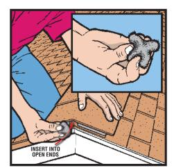
**7.** To close off ends of vent, fold over a section of End Plug material (2 per ctn.) and pinch together (see inset). Insert End Plug material between vent legs. Once seated properly, seal in place with flexible caulk.
