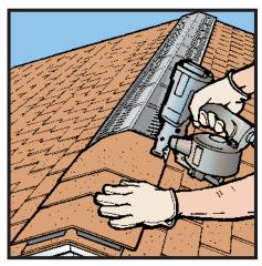
**6.** Center shingle cap on vent and nail along "NAIL HERE" guideline. Continue applying caps until all vent is covered with ridge caps. Do not overdrive nails. Nail head should be flush with top of shingle, without indenting it. Pre-forming caps in cold weather helps avoid cracking.
