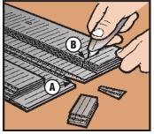
2. Use a utility knife to cut out a "V" shaped notch from the centerline approximately 13/4" in from edge and remove loose material (A). Cut through the bottom 3 layers of the vent as pictured (B) (located approx. 13/4" from & parallel to the end). Remove loose pieces. Be careful not to cut into top layer.
